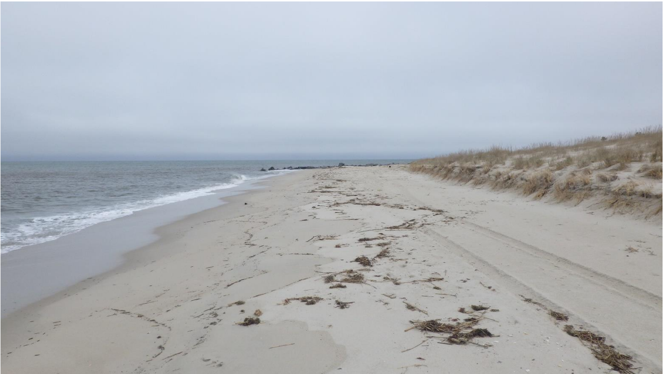
Figure 18. The April 2, 2026 photo (view to the northwest from the CMP-8 profile) shows the extent of wave runup onto the berm, foreshore, and Alexander Avenue groin. An erosional scarp along the dune toe shows the extent of past exposure to waves, though the dune field continued to grow over 2025-2026.
