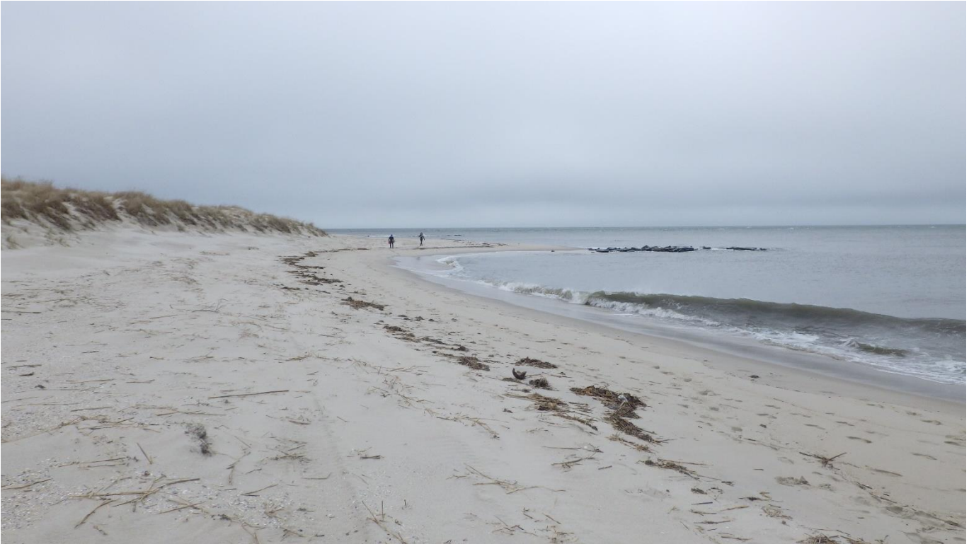
Figure 16. The April 2, 2026 photo (view to southeast) at profile CMP-7 shows the berm crest, foreshore, and exposed Pearl Avenue groin. The foredune continued to grow seaward over 2025-2026; evidence that there is ample natural sand transport to this groin cell.
