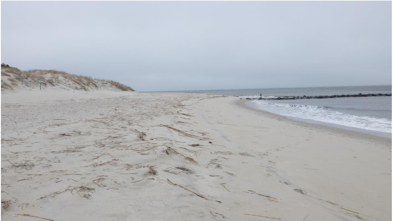
Figure 12. The April 2, 2026 view to the southeast from profile CMP-5 shows the dune, berm crest, foreshore, and the Surf Avenue groin. The dry beach landward of the “Beachsaver” unit was less than 100 ft in width.
