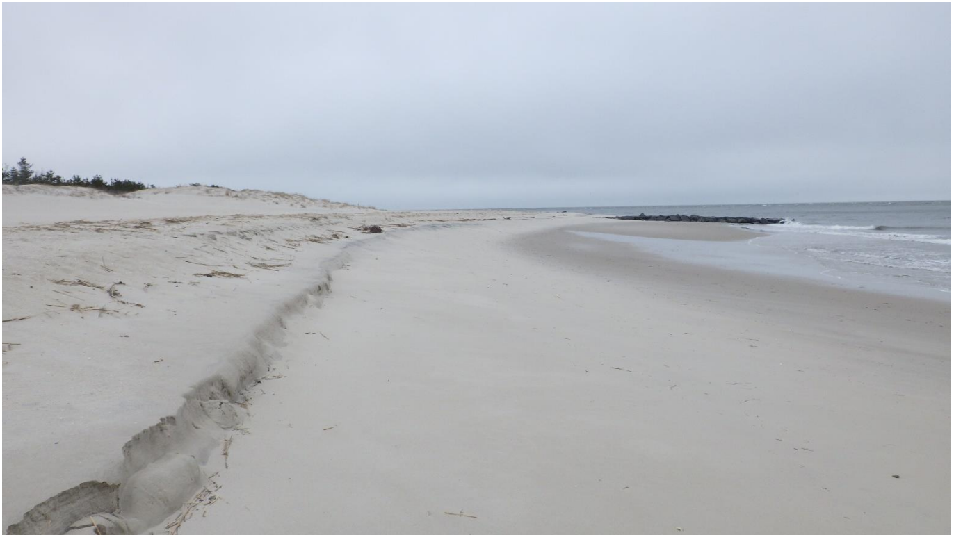
Figure 10. The April 2, 2026 photo at profile CMP-4 shows the conditions of the berm crest and scarp that resulted from higher waves during a full moon. The Coral Avenue groin appears within the swash area of the profile. The backshore elevation adjacent to the dune toe was higher than measured in the April 2025 survey.
